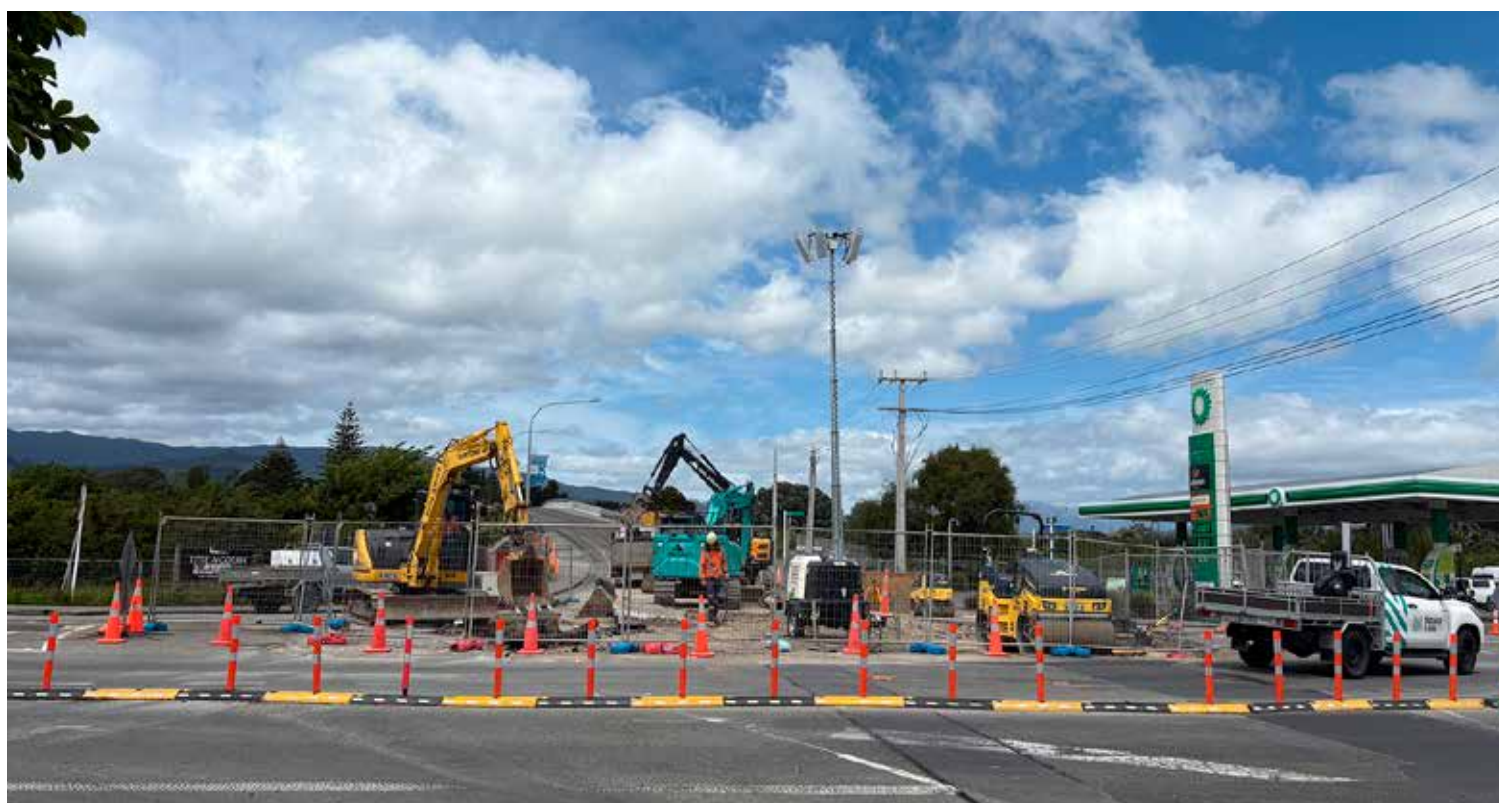
Recent work at the BP roundabout at the intersection of Mill Road and old State Highway 1.
